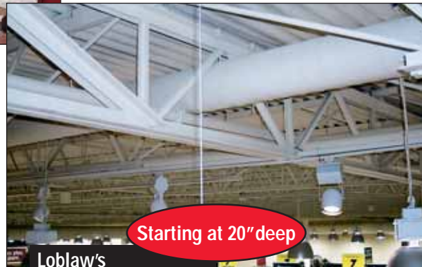
Loblaw's St. Georges, Quebec Joist girders
